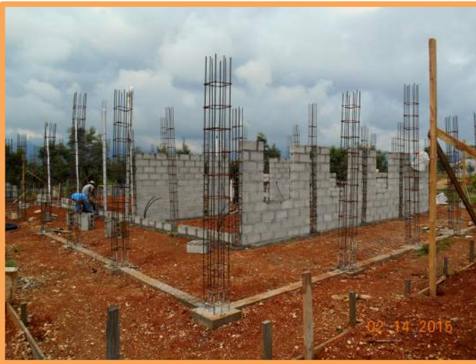
The second home / administration building's walls are UP!
