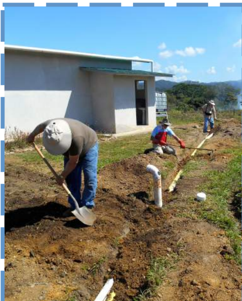
Ditches were dug, pipes placed and the ditches filled in.
