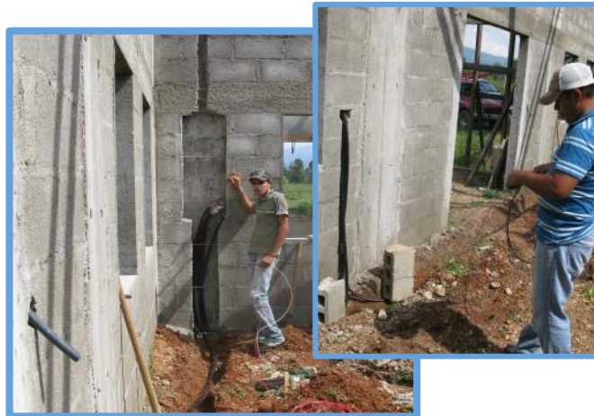
Electrical wiring being installed.
